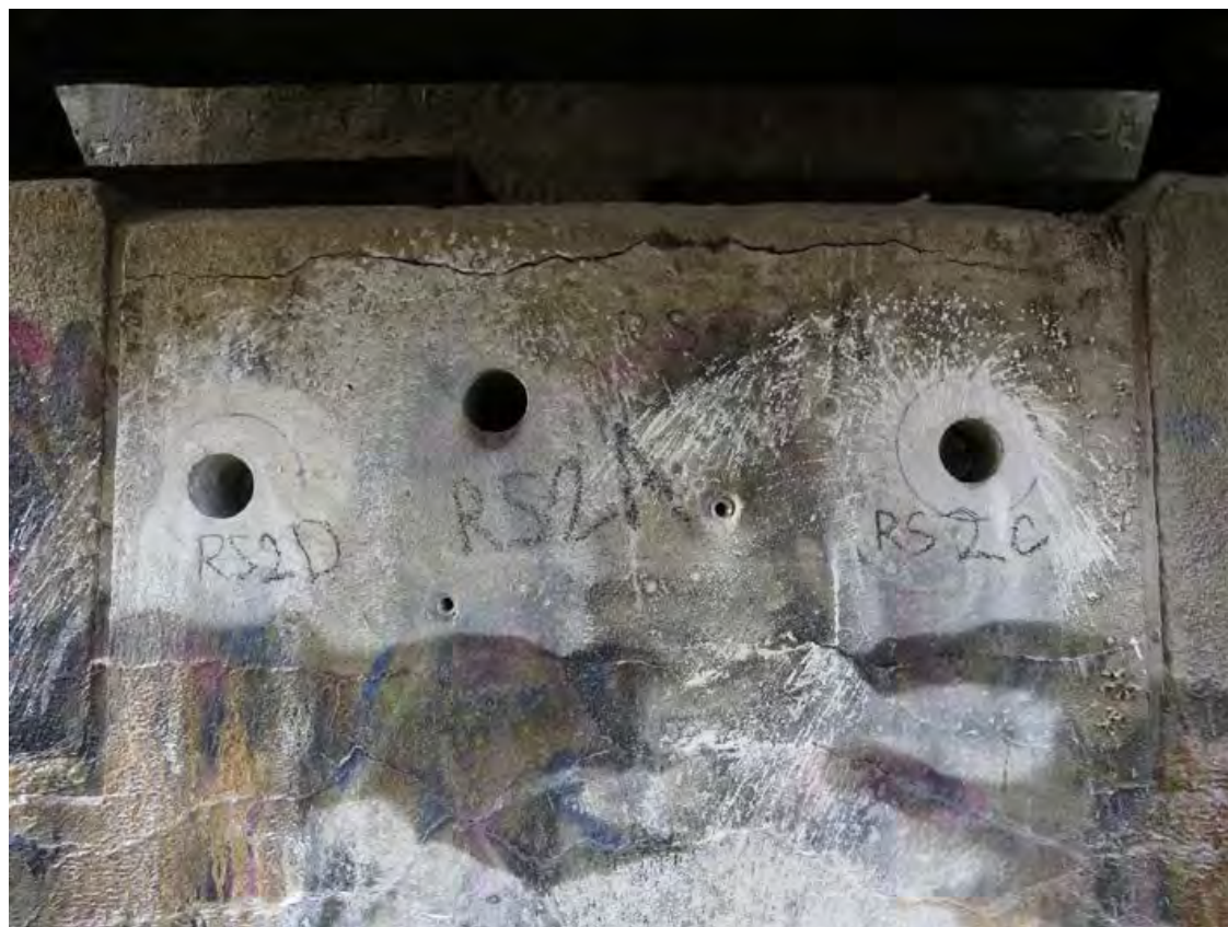
Fig. 2 The place where the specimens RS2-D, RS2-A, RS2-C were taken from the bridge abutment – a location with PRC (November 2019).
