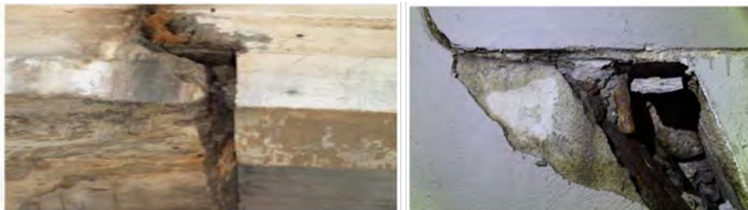
Fig. 1 Dapped end beam and corbel corrosion: Granada, Spain (left) and M-30, Madrid (right) [1]
