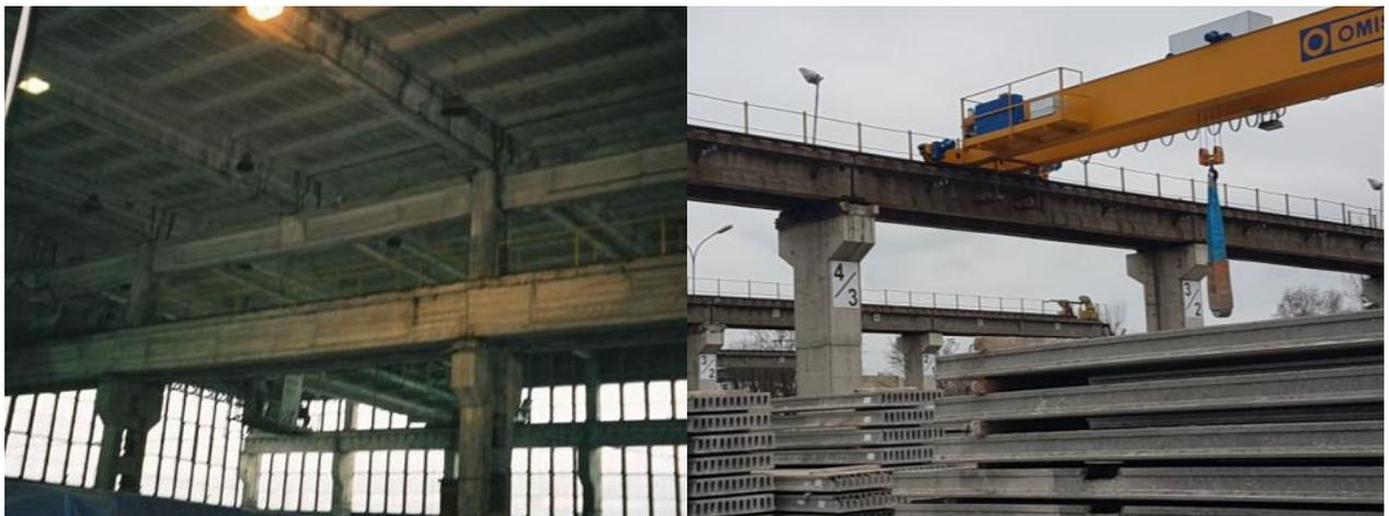
Fig. 1 Post-tensioned beam track for the overhead cranes inside the industrial plant (left) and external post-tensioned beam track for the overhead cranes (right).
